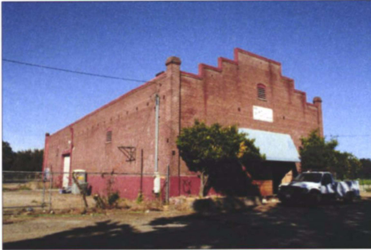
Figure C: Elk Grove Winery warehouse, view facing northwest (GPA, September 2018)
